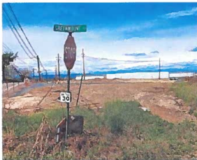
A major project is happening along Greenmount Road just north of the Pennsylvania-Maryland line in Antrim Township to improve infrastructure. It also includes the development of a warehousing and logistics facility, seen in the background.
