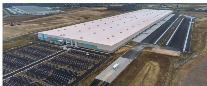
Walmart DC / Exit 24 Southampton Township
